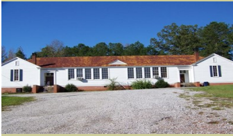
Woodworking Education Center 10544 Hwy 17, Maylene, AL 35114
